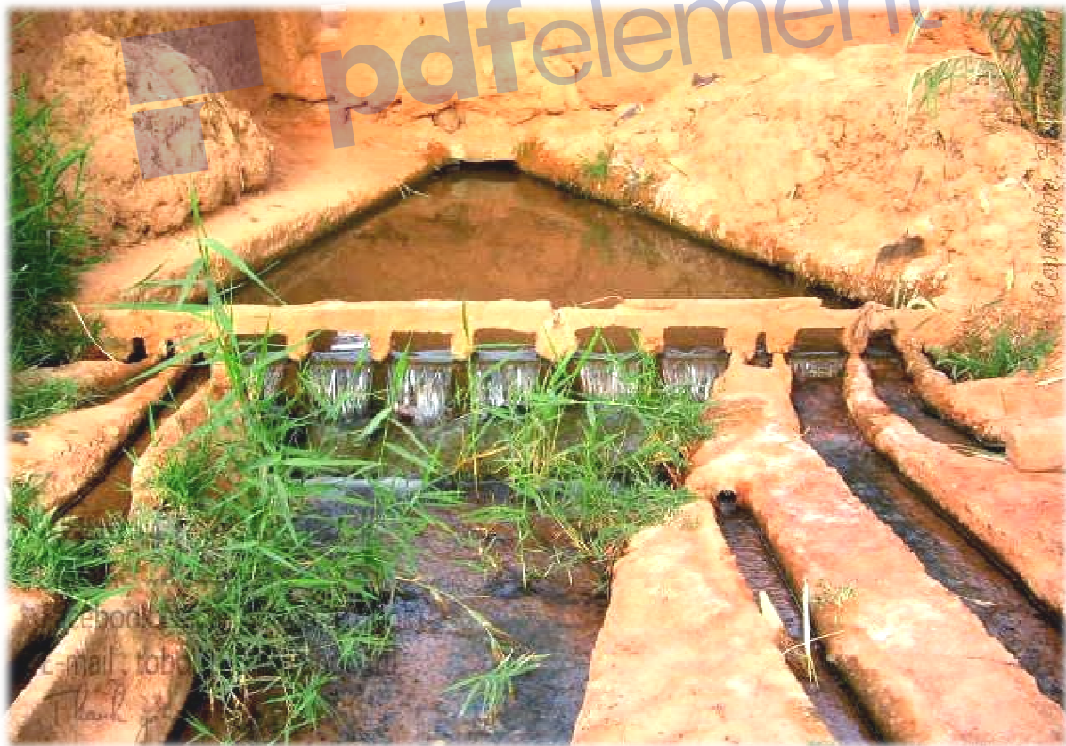
Figure. 02: Kasriya, Fggara: Water distribution system for irrigation
