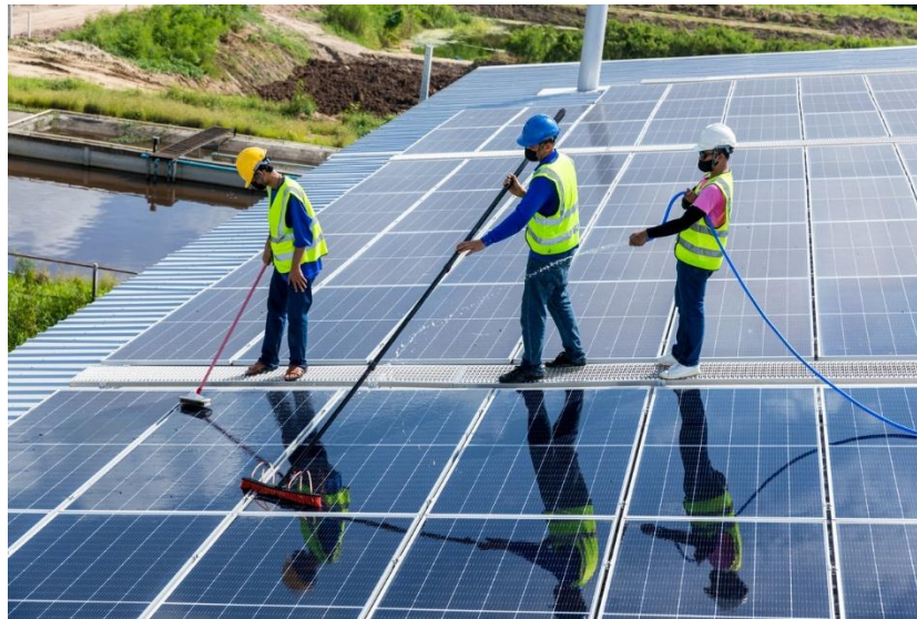
Figure 15: Manual solar panel cleaning workers [19]
