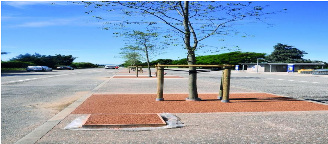
Figure 7-I: Parking en béton drainant.
