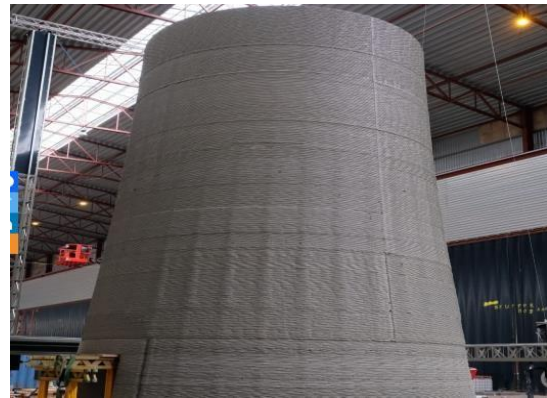
figure II.19 : Le mât béton
