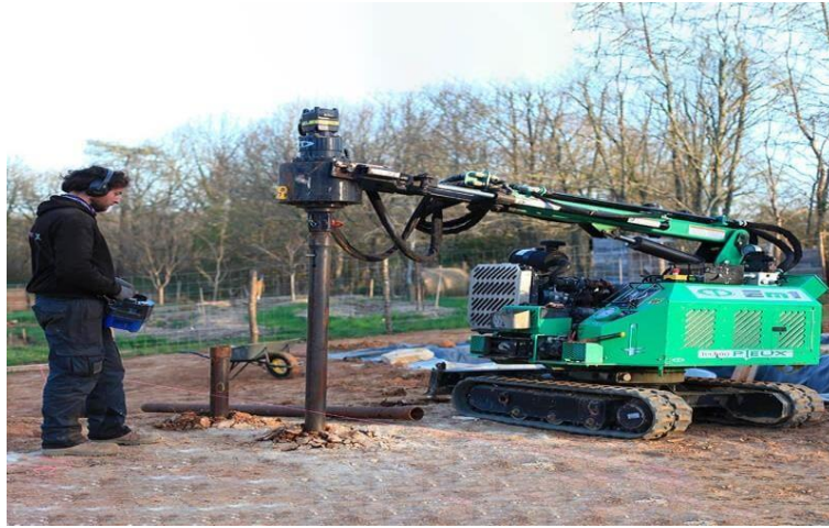
Figure III.11: Ancrage Des pieux vissés
