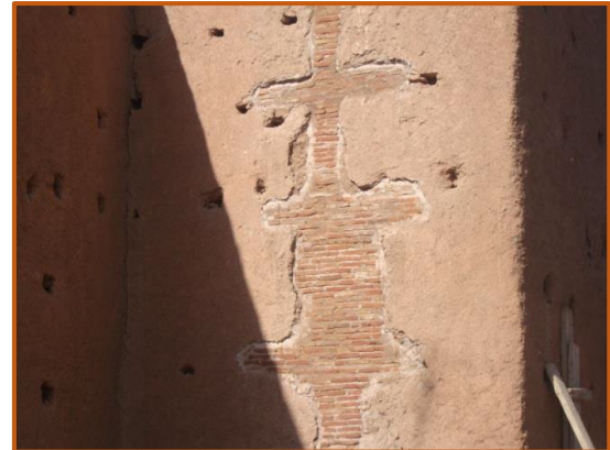
Figure 172 : Colmatage Finition.
