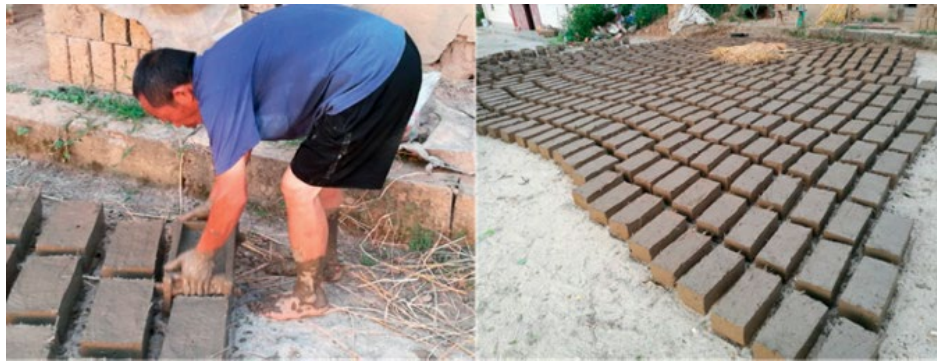
Figure. 2.1. Production Method of Molded Adobe Bricks [32].
