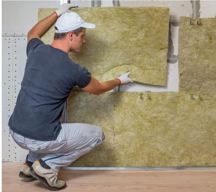
Figure. 2.2. Mineral wool used as thermal insulating into building.
