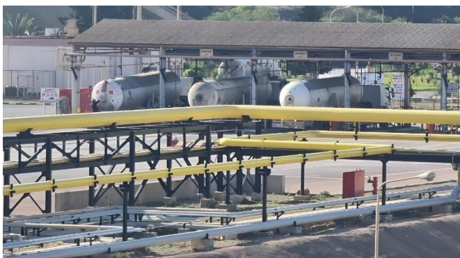
Figure I. 9: Section chargement camions
