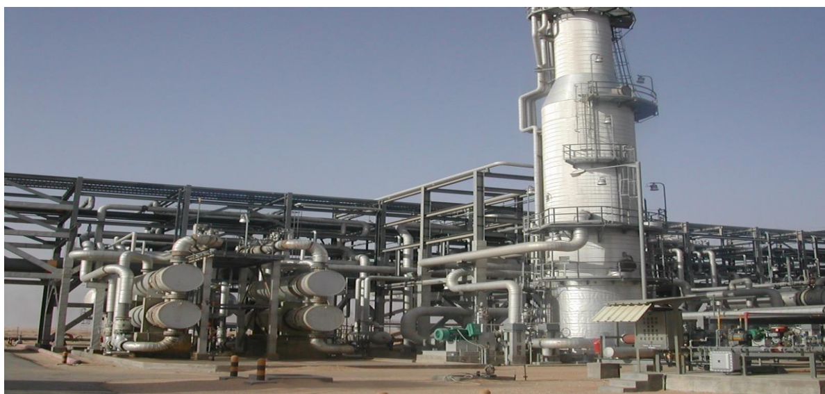
Figure I. 4: Section stabilisation haute pression.
