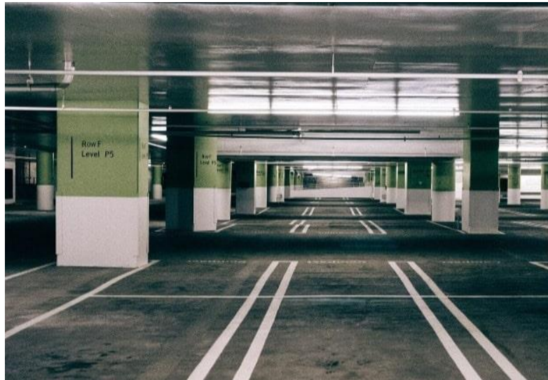
Figure 1. 3. Exemple de parking souterrain. [2].
