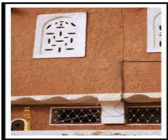
Fig80- fenetre - Source (fondation Amidoul,2006)
