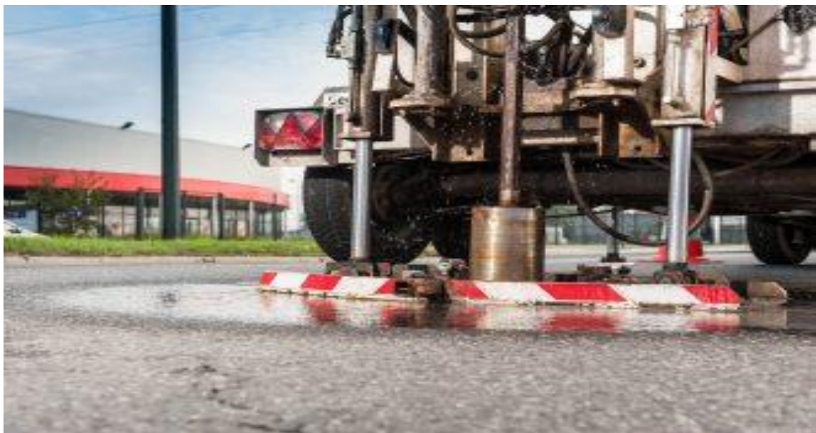
Figure II.7 : Le carottage
