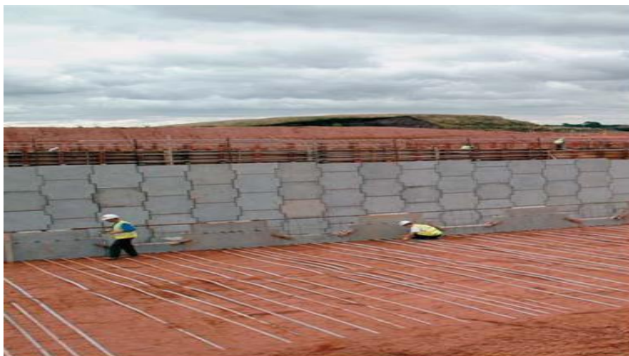
Figure 2.18: Disposition des armatures de renforcement
