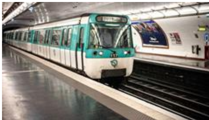
Figure 27 Station Sully Morland Métro Paris Ligne 7
