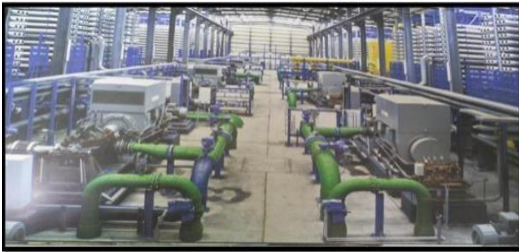
Figure II.9 : Osmose inverse (Station de MOSTAGANEM)
