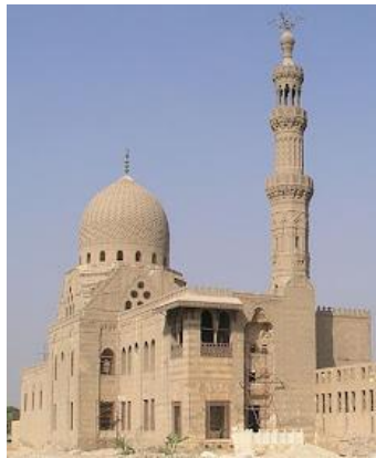
Figure 8 mosquée Baybars Egypt
