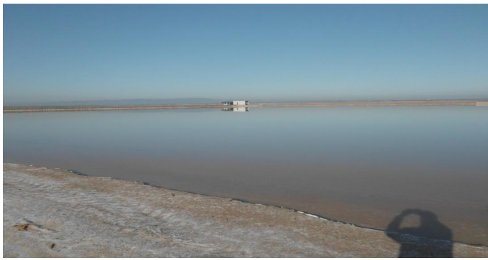
Figure 09 : Station de pompage.
