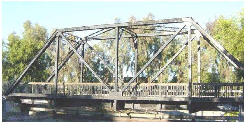
Figure 22: pont en treillis
