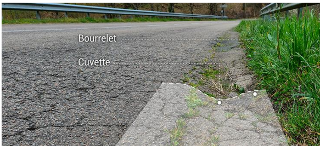
Figure I.5: affaissement
