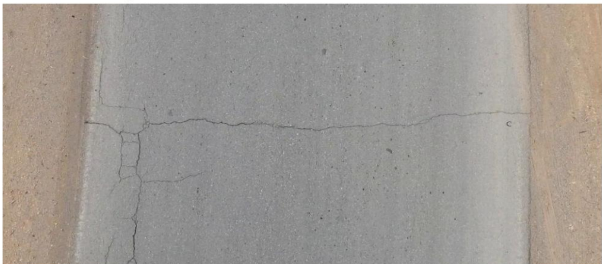
Figure I.3: fissure transversal
