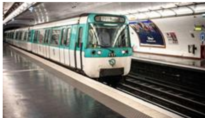
Figure 26 Station Sully Morland Métro Paris Ligne 7
