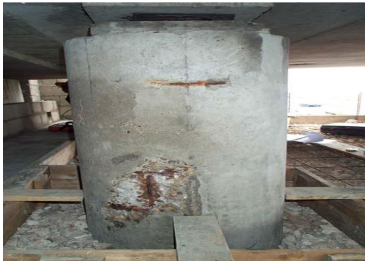
Figure 3.7: pile de pont.
