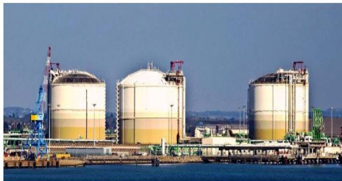
Figure I-2: Bacs de stockage.
