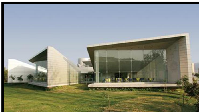
Figure II.27: vue de face du restaurant. (A. Ramprasad Naidu, Archdaily).
