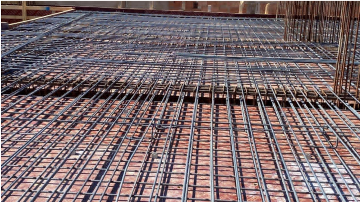
FIGURE 9 : Plancher dalle pleine
