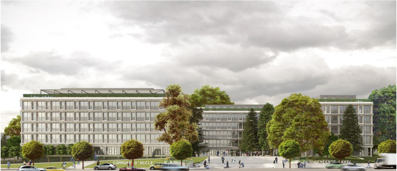
Figure 46 : la façade principale
