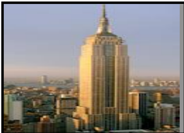
Figure 3 : l'empire State building
