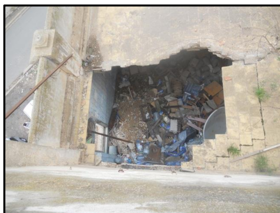
Figure 126: Un plancher effondré (bain maure) 112
