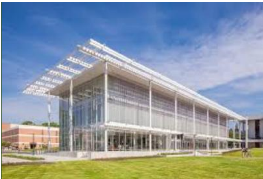
Figure 40: Watt family innovation Center (Source: Jonathan & Michelle, Archidaily, 2016)
