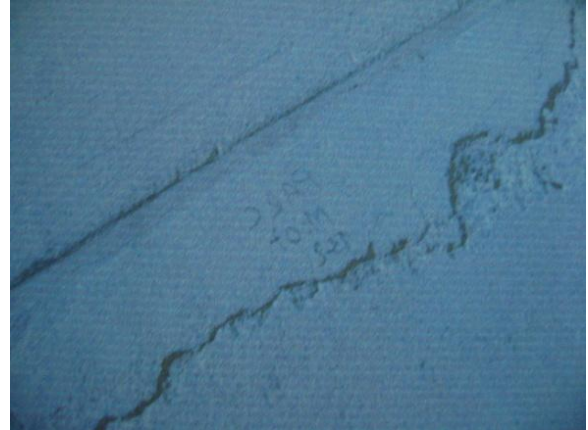
Figure 4.28 : Epaufrure graves (parking)
