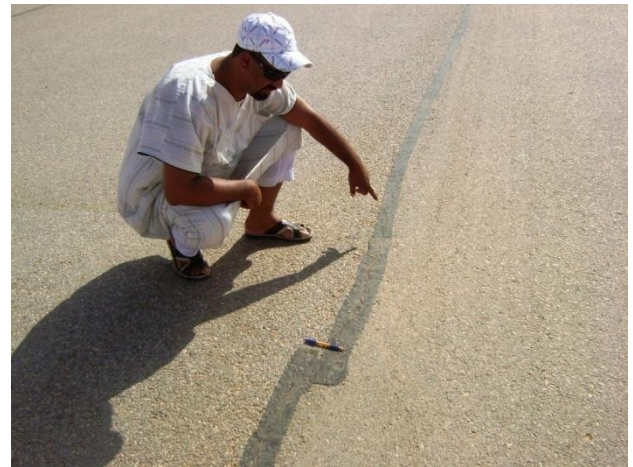
Figure 4.7 : Fissure de joint
