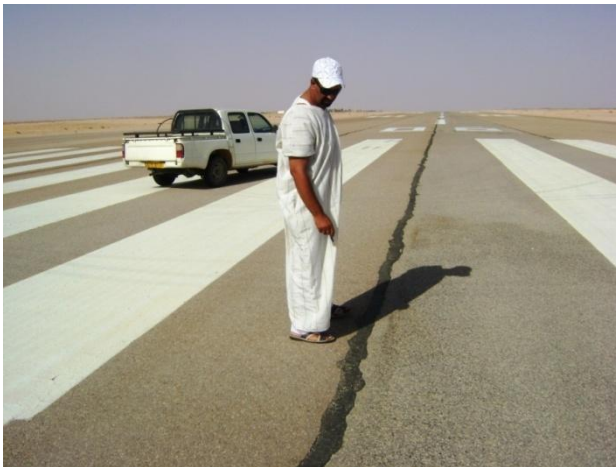
Figure 4.7 : Fissure de joint
