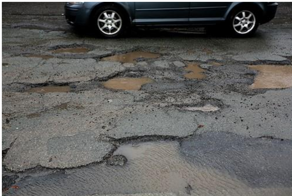
Figure II.1 : Arrachement
