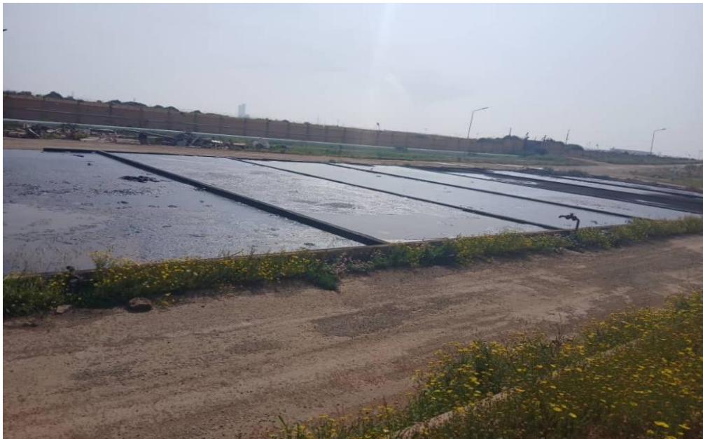
Figure II.12: Sludge dewatering unit of Unit 1800.
