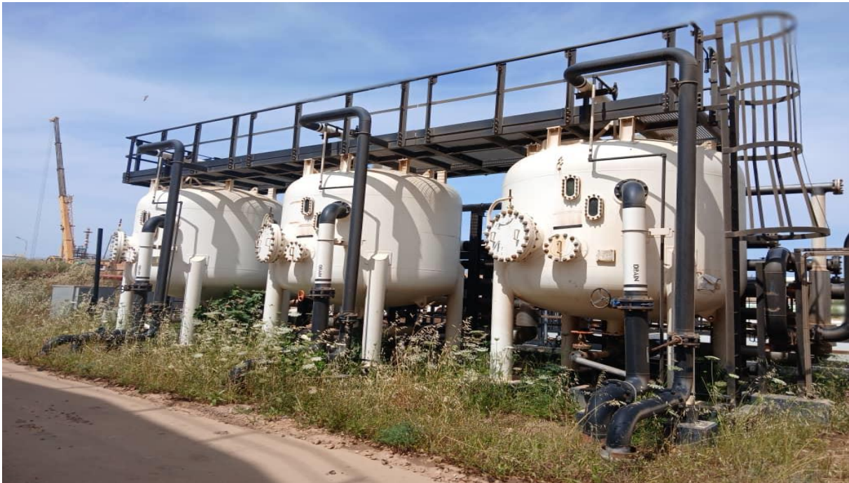
Figure II.19: Sand filters of Zone 27
