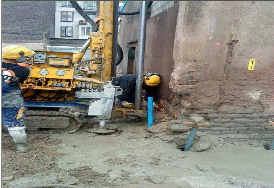
Figure III.11 : Technique d'injection
