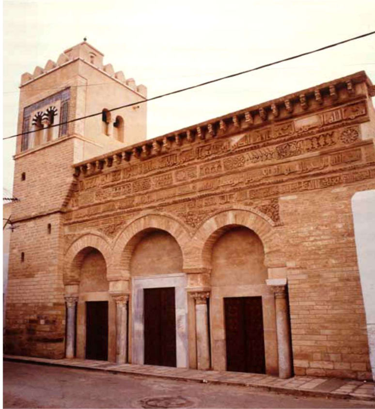
Figure 14 : Mosquée Ibn Khayroun (post restauration)
