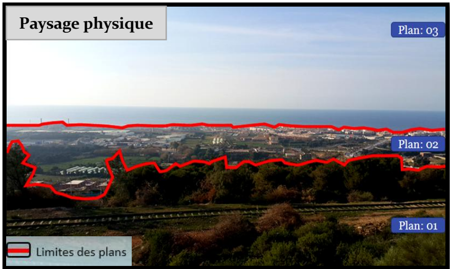
Figure 33: Photo de constats
