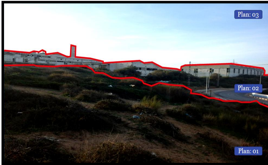
Figure 37: Photo de constats
