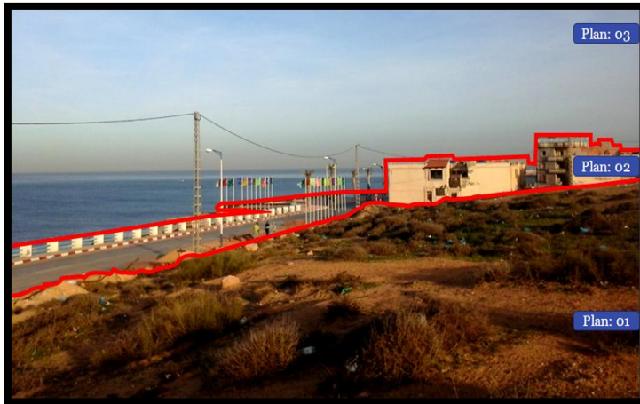
Figure 35: Photo de constats
