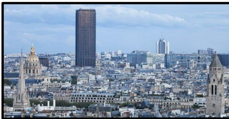
Figure 03 : la tour Montparnasse, Paris, France
