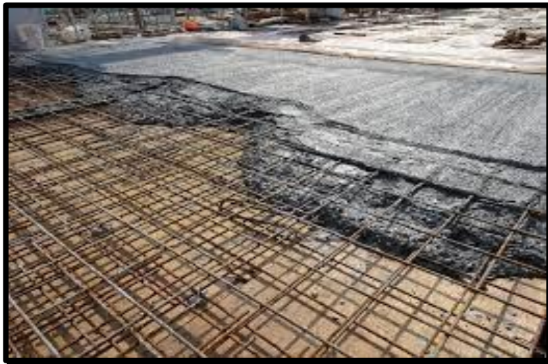
Figure I.6: Plancher en dalle pleine
