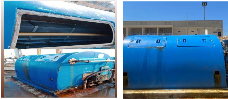
Figure 31: Les Tamis fins rotatifs TBS (Travelling band screen).
