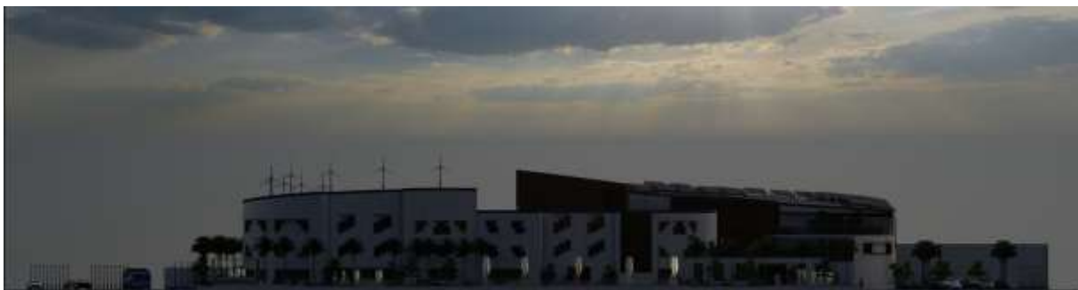
Figure 77 : Façade secondary (source: Auteurs)
