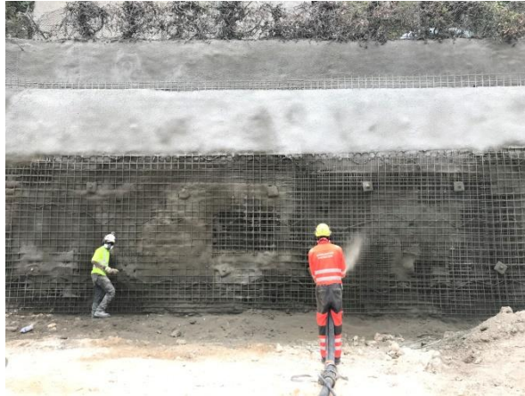
Figure I.1.2 : La projection de coulis de ciment [3]
