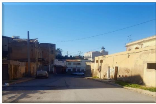
Figure 69: photo de site
