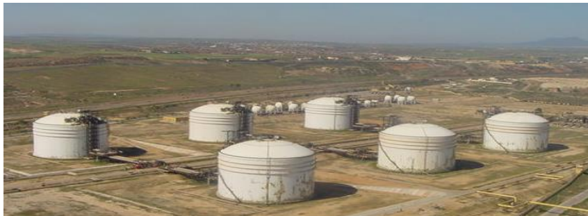
Figure I.6 bacs de stockage
